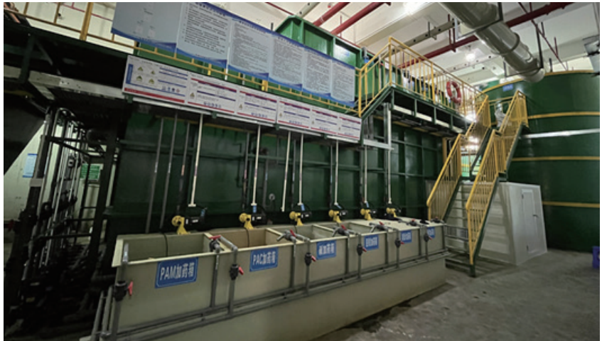
Expansion of wastewater treatment equipment
